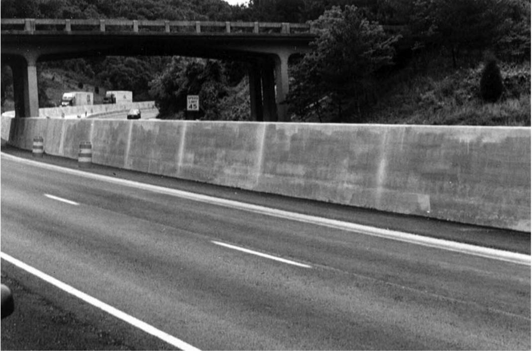
**Figure 15.7** Single-Slope Concrete Median Barrier
