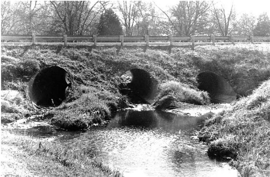
(a) Corrugated metal arch culvert (ARMCO)
