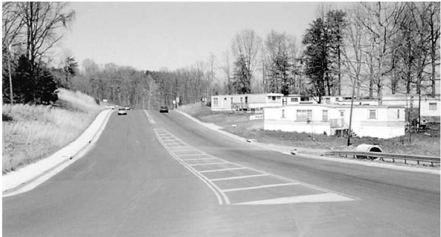
(b) Island formed by pavement markings (flushed island)
