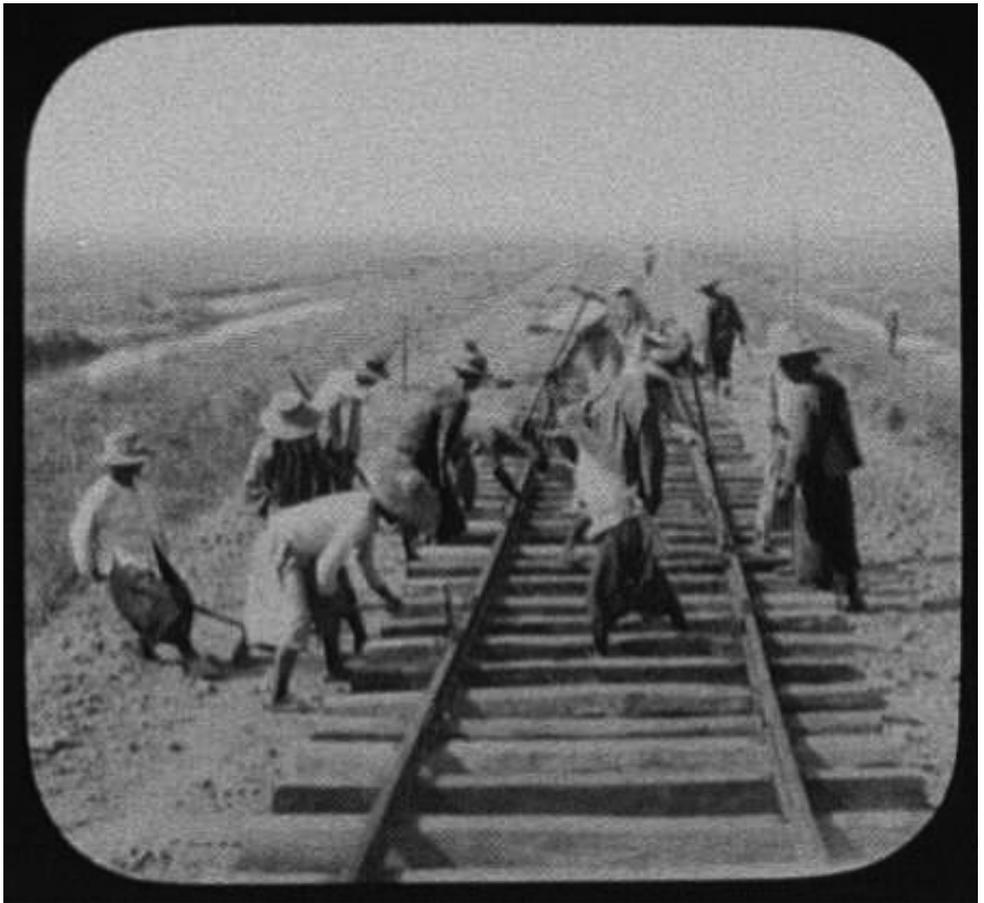
**Figure 1.2** Workmen Repairing Railroad Track—1895
