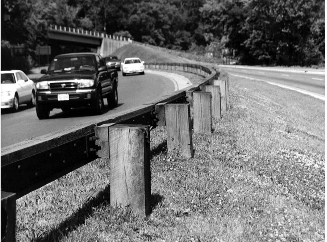
**Figure 15.6** Steel-Backed Timber Guardrail
